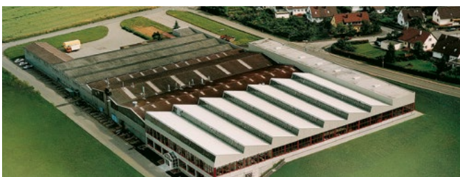
Häfele Production Plant Jettingen, Germany
